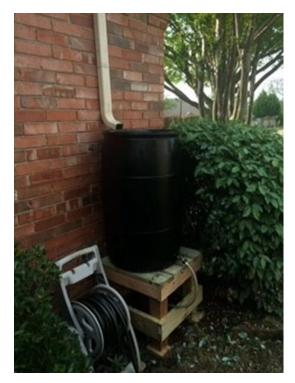
You can build or purchase your rain barrel. If you choose to build you will need a few supplies: food grade barrel, insect netting, faucet, 1.75 in. bulkhead fitting (internal pipe threading), drill, jig saw, silicone caulk, teflon tape. The Texas A&M Agrilife Research Extension in Dallas has excellent instructions on building rain barrels.
